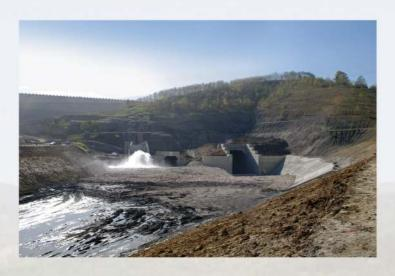
Dam type Rockfill dam with clay core Dam height 78 m 838 m Crest length Crest width 12 m Foundation width 430 m Morning glory 1,010 m³/sec 59 m L\*7.5 m Dia Spillway type Spillway discharge Spillway shaft dimensions 370 m L\*7.5 m Dia Spillway tunnel dimensions **Diversion tunnel dimensions**
